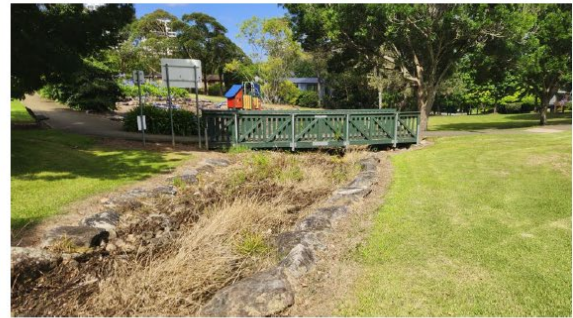
Downstream watercourse with rock stabilised banks
