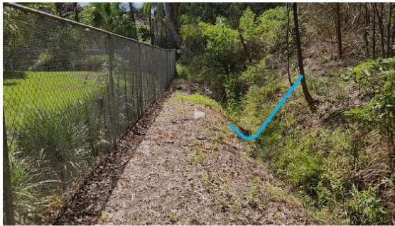
Confined, stable watercourse channel + steep vegetated bank
