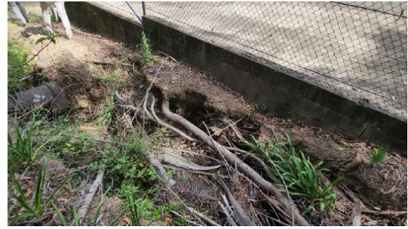
Erosion of creek channel caused by undercutting of bank
