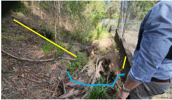
Steep banks on LHS, Property retaining walls on RHS
